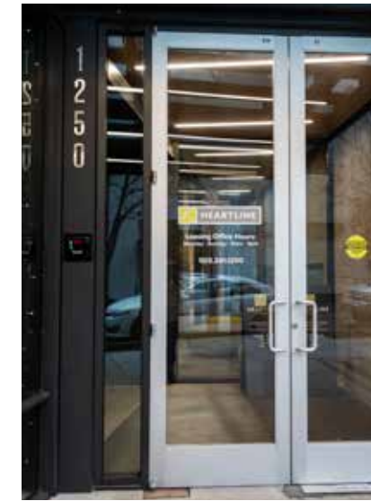
Entrance vinyl & building numbers
